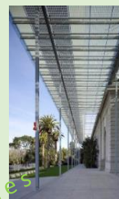
Ombrières PV, San Francisco, USA
